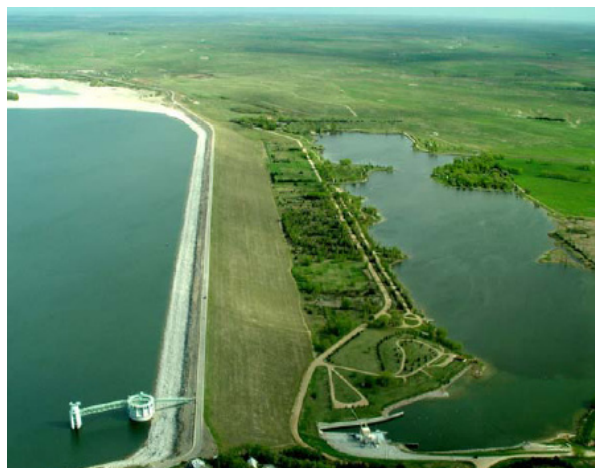
Kingsley Dam on North Platte River, completed in 1941, directly controls flows downstream through central Platte River. Photo by W.L. Graf, May 2003 (NRC 2004).
